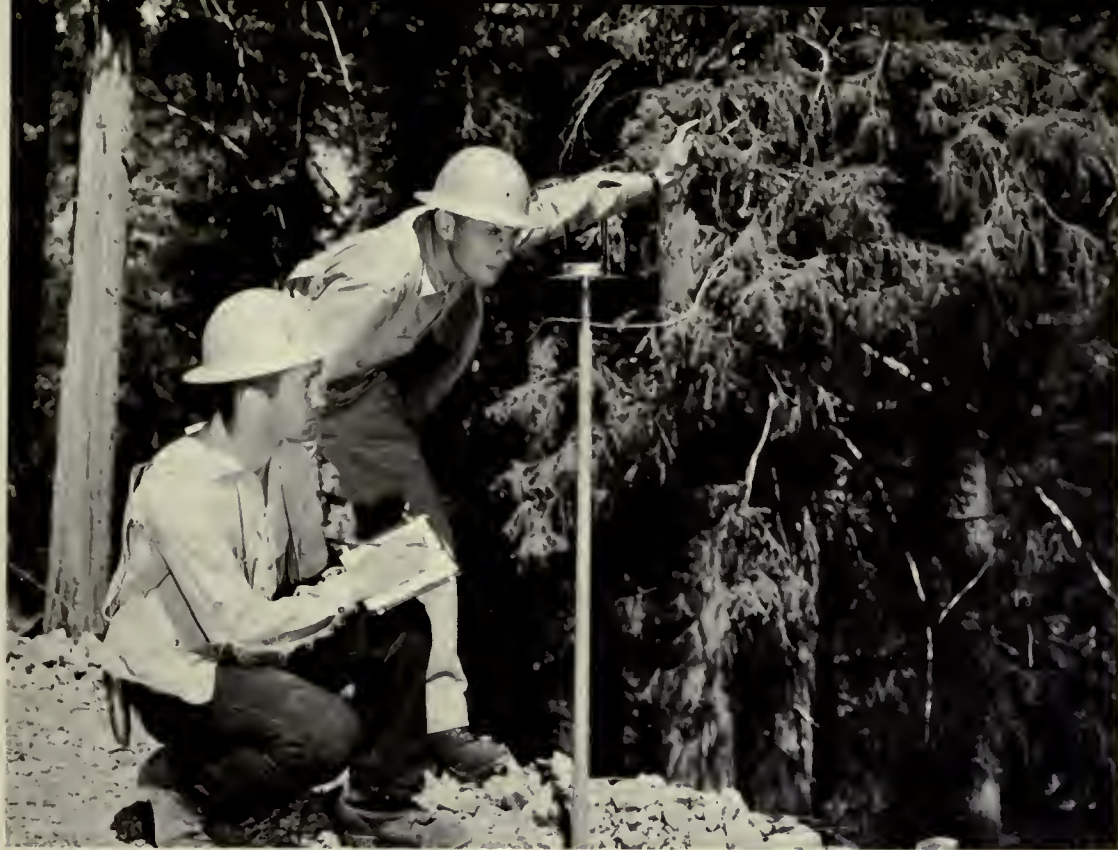
A public land access road takes shape as a Bureau of Land Management engineering team runs a preliminary survey.
